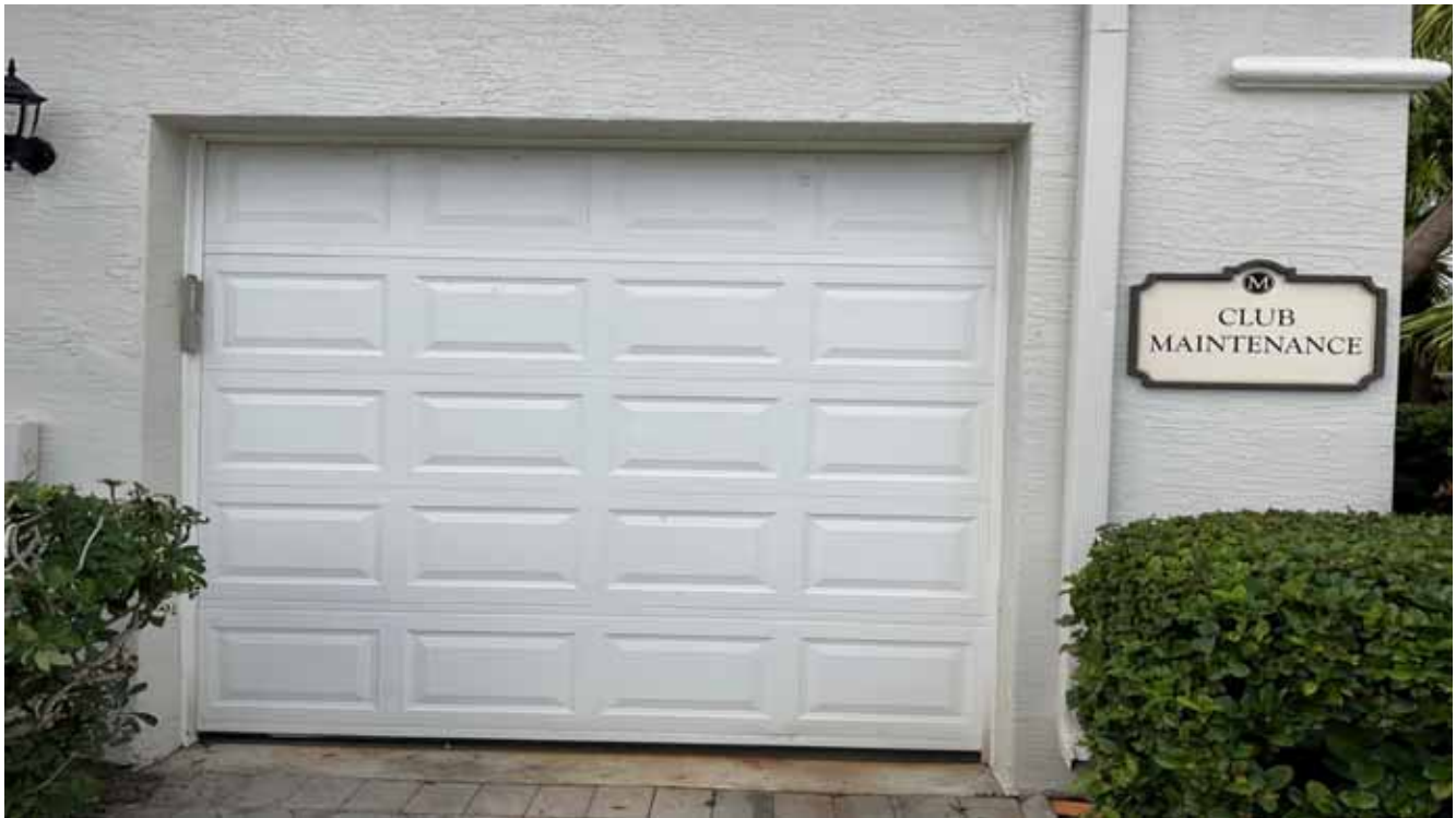
Clubhouse - Maintenance Area
