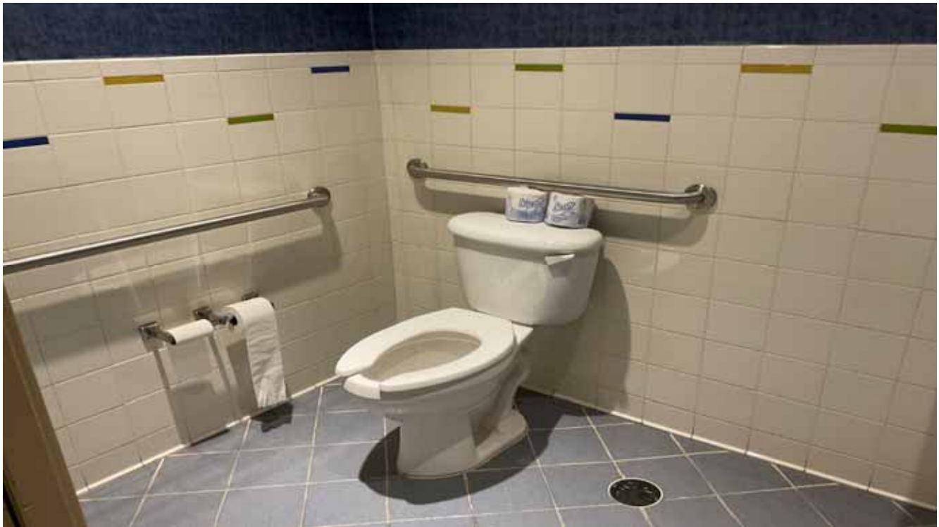
Clubhouse - Kid's Club Boy's Restroom
