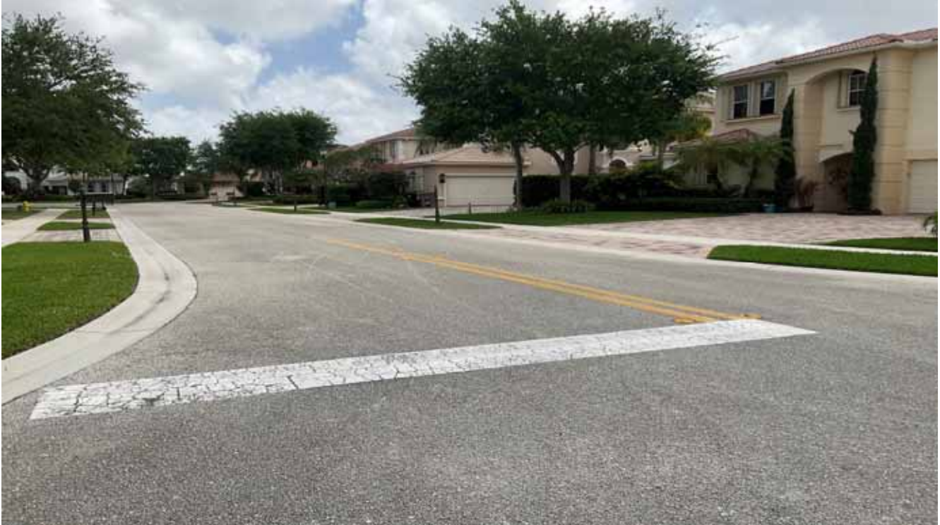
Pavement, Asphalt Road - Alegria Way
