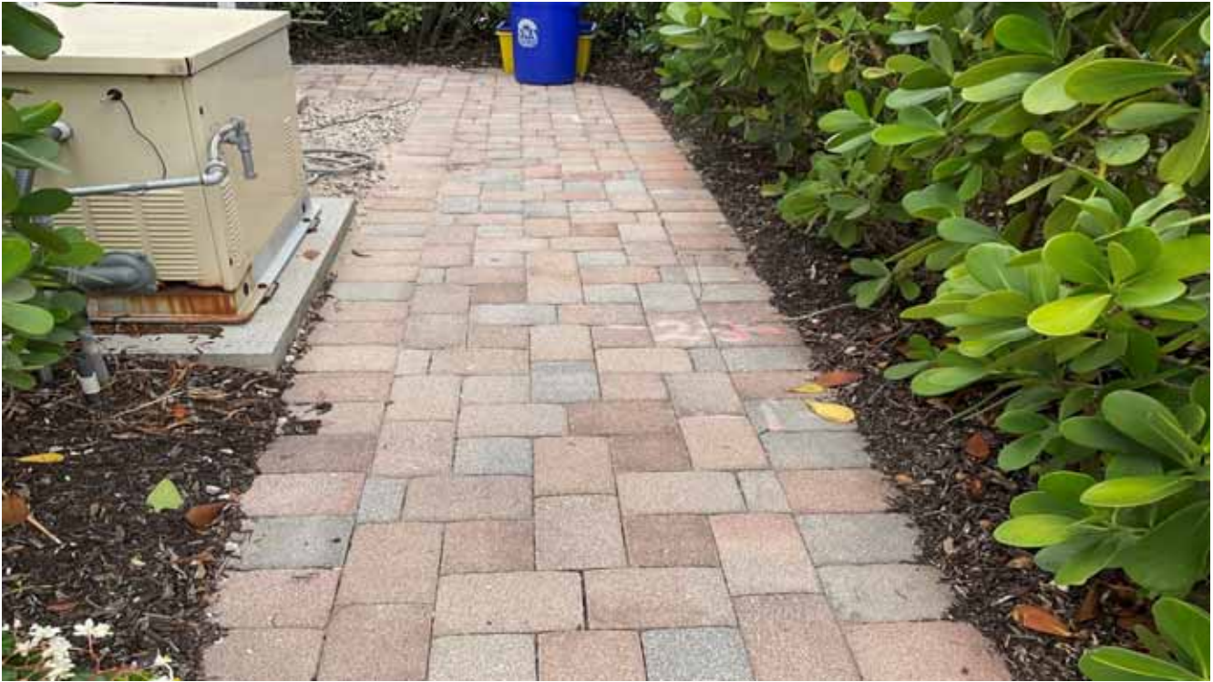
Pavement, Pavers Sidewalk - Gatehouse
