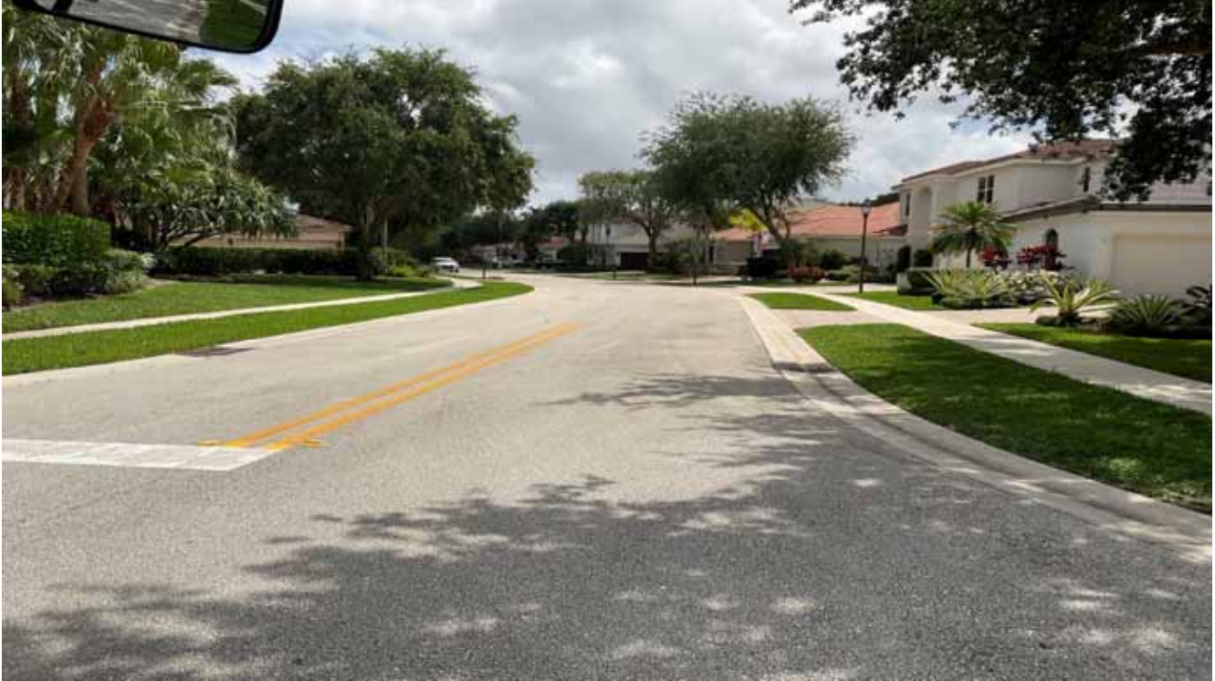
Pavement, Asphalt Road - Villa Nueva Place
