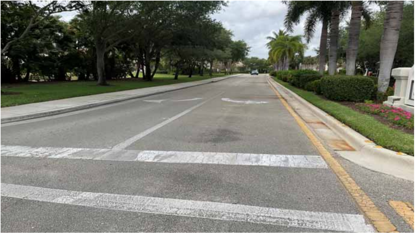
Pavement, Asphalt Road - Sedona Way
