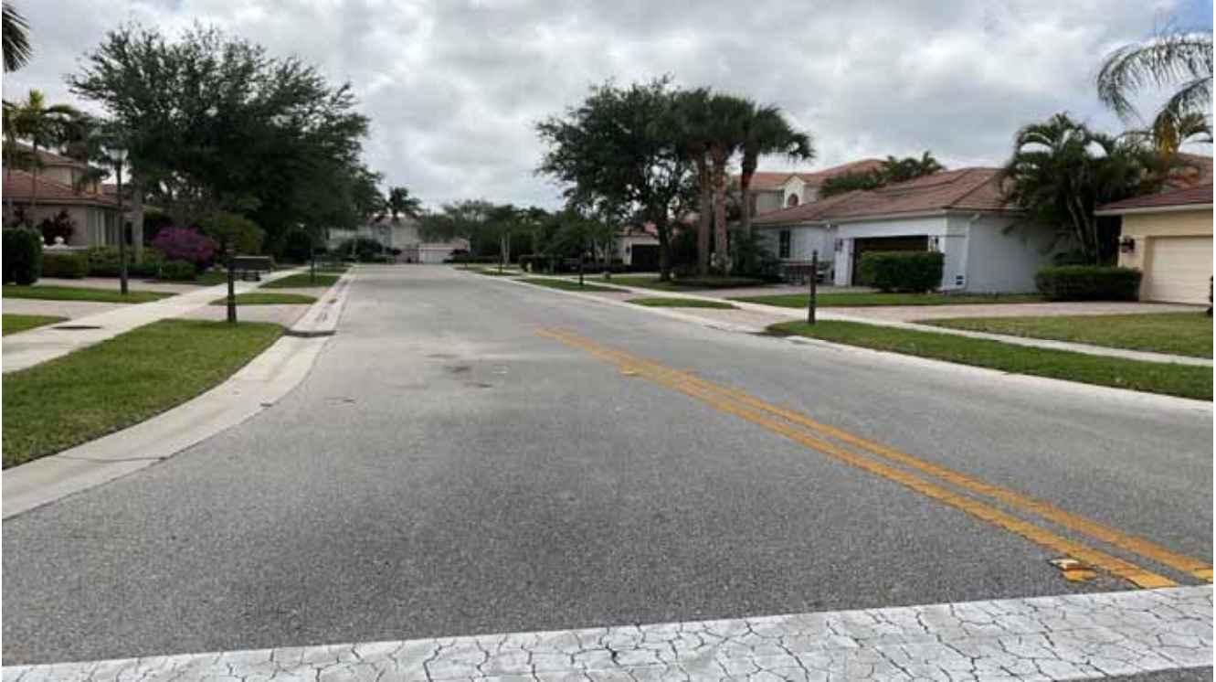
Pavement, Asphalt Road - La Vida Court
