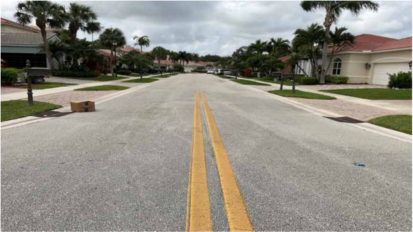
Pavement, Asphalt Road - Casa Grande Court
