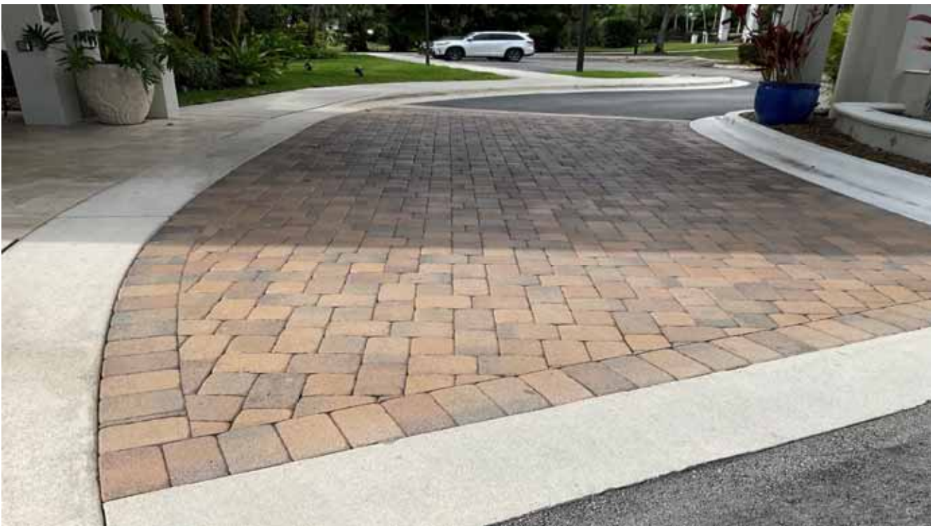
Pavement, Paver Parking Lot - Clubhouse
