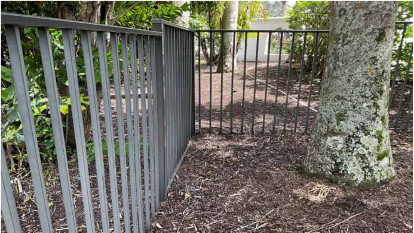
Entry Fence - Neighborhood
