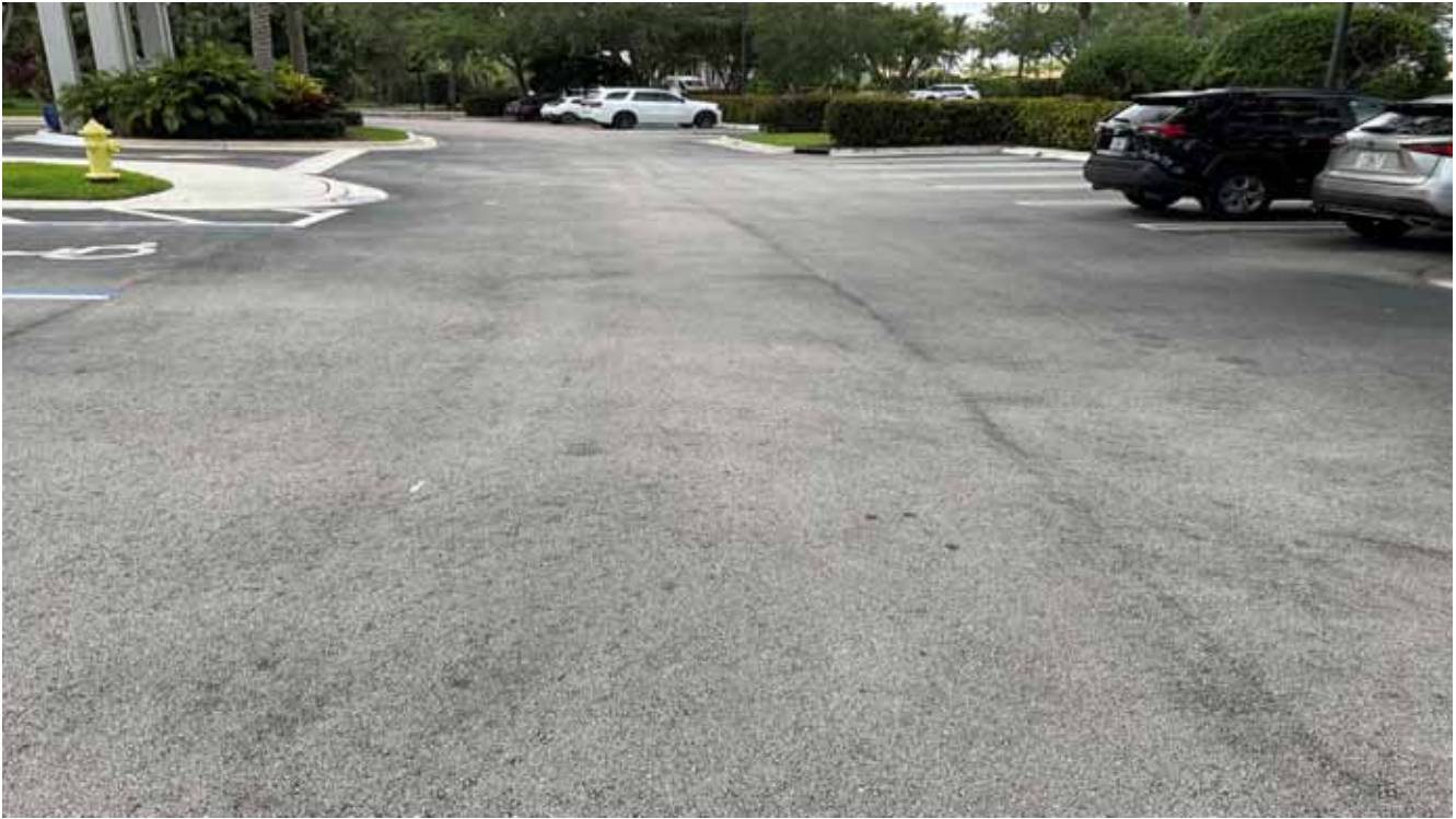
Pavement, Asphalt Parking Lot - Clubhouse
