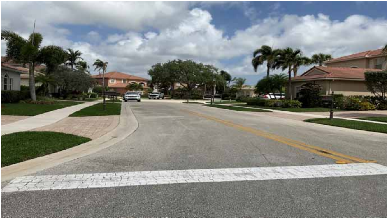
Pavement, Asphalt Road - Via Escobar Place
