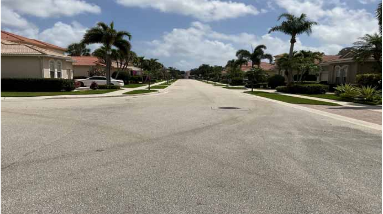
Pavement, Asphalt Road - Via Condado Way
