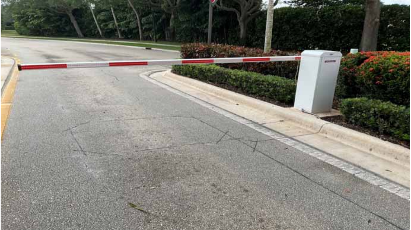
Vehicular Gate Operator - Gatehouse
