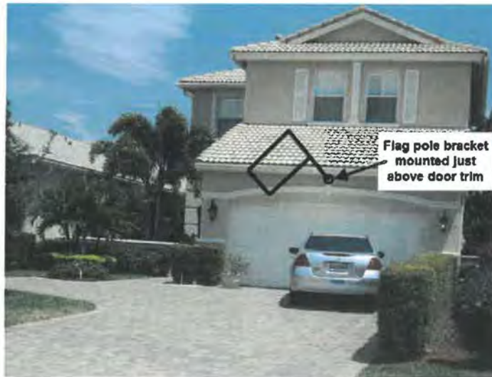
Isle Verde 2-story house front load garage (Acceptable flag pole bracket location)
