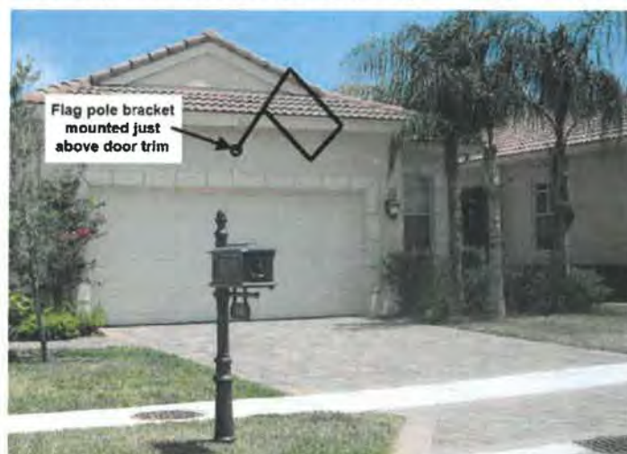
Isle Verde 1-story house (Acceptable flag pole bracket location)
