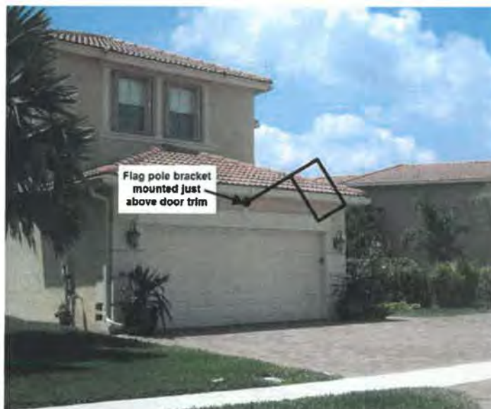
Isle Verde 2-story house front load garage (Acceptable flag pole bracket location)
