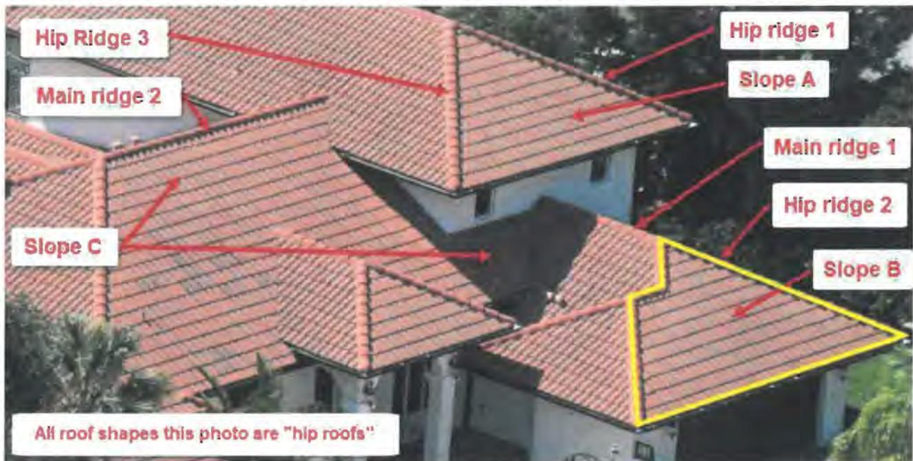
Roof slopes and ridges defined
